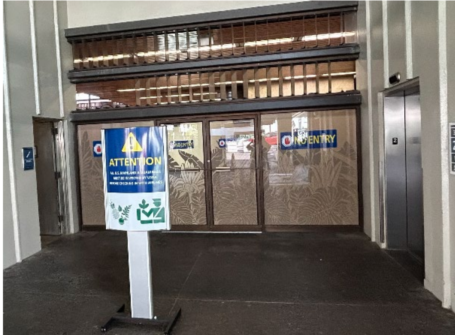
Lobby 6 Swing Doors
